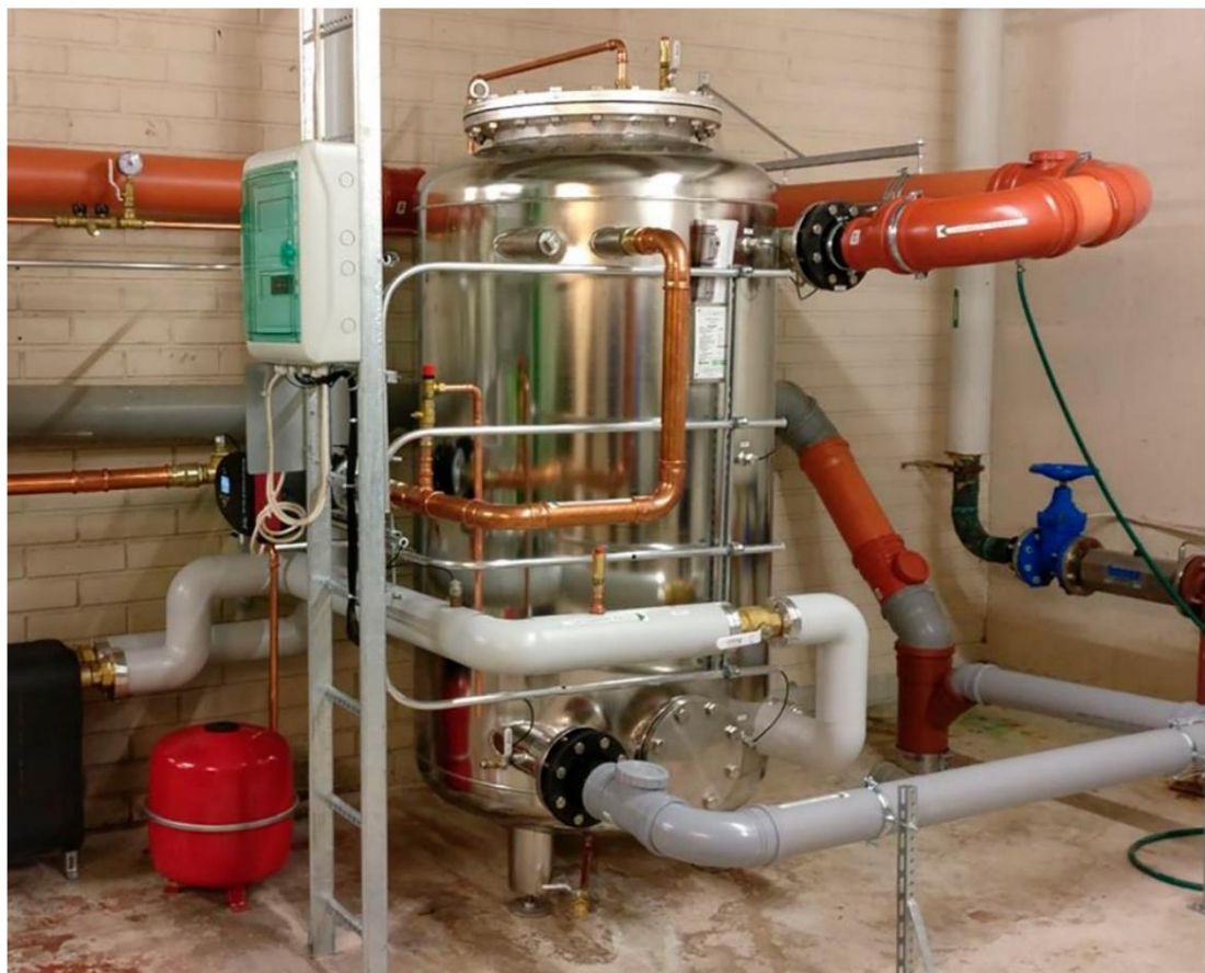
Figure 10. Kokkola Swimming Pool Vesiveijari's waste water heat recovery system ( https://www.ecowec.com/uimahallit-ja-kylylat/uintikeskus-vesiveijari-kokkola/ )
